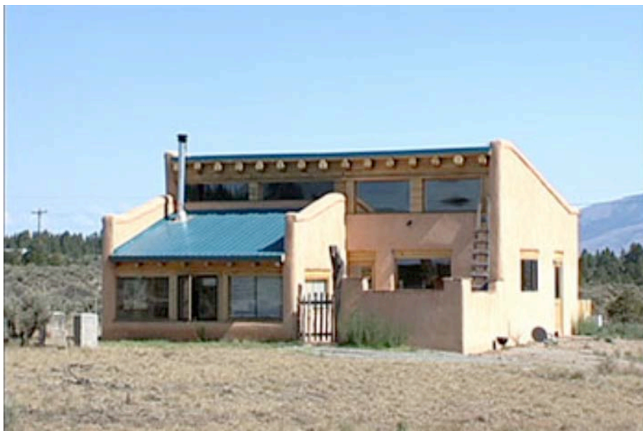
Figure 7 Passive Solar Guest House
